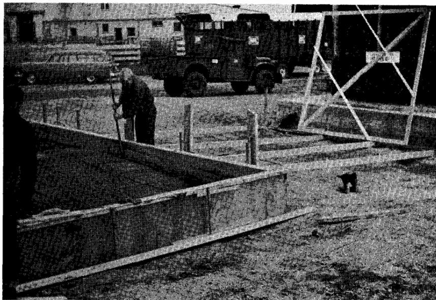
Pouring concrete for a floating slab as a base for a 16' x 40' concrete stave silo. Two layers of reinforcing rod were used.
